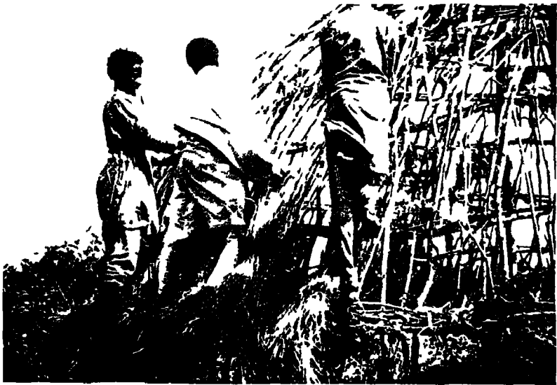
The roof is thatched over a frame of poles tied together with leather.
