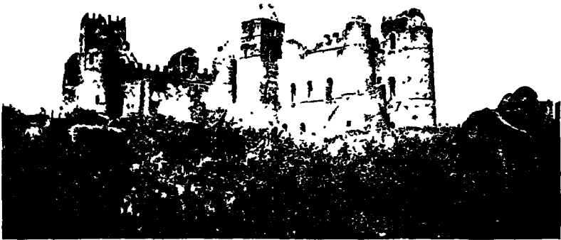
Fasil's palaces at Gondar.
